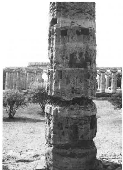
A detail of a column of the Temple of Neptune showing the borings of marine molluscs. — Photo: Marita Ahlström.
