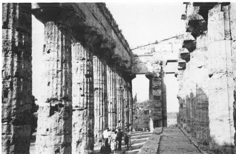
The columns of the S.C. Temple of Neptune, Paestum. Showing the typical effect of marine erosion with miniature caves up to 5 feet. — Photo: Marita Ahlström.
