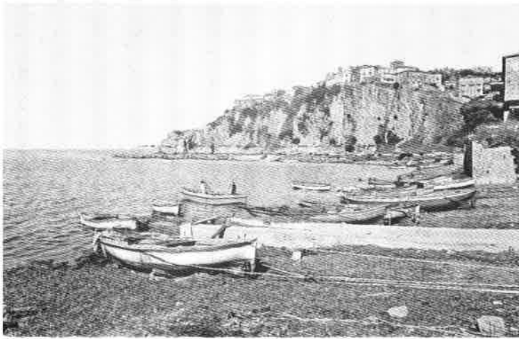
At Agropoli, 10 km south of Paestum. The rock is marked by marine erosion along the line indicated: the same as that of the temples.
